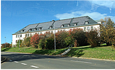
Solar panels on a building at the US Army garrison in Baumholder
